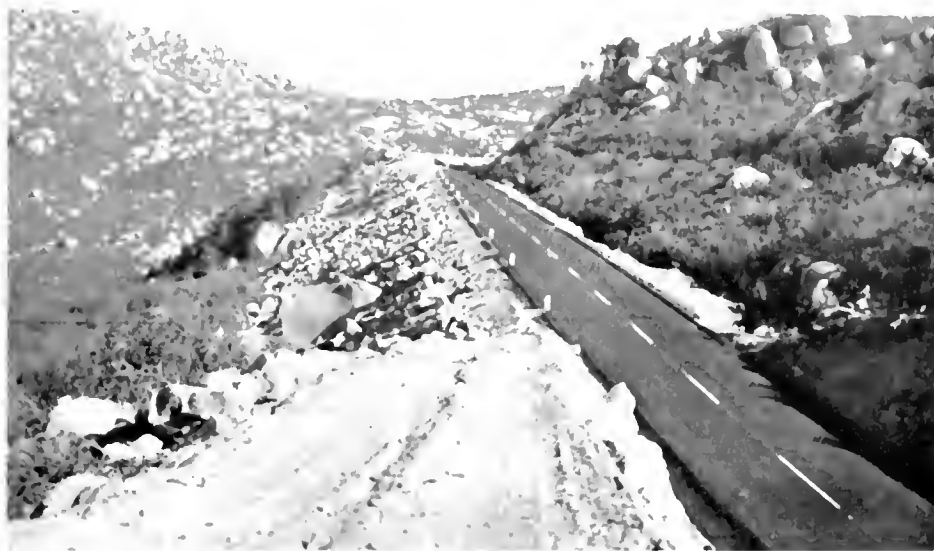
Mile and a half stretch of 7 per cent grade on new highway through boulder covered hills
